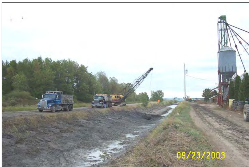
Excavated sediment and soils being trucked off-site during a drain reconstruction project.
