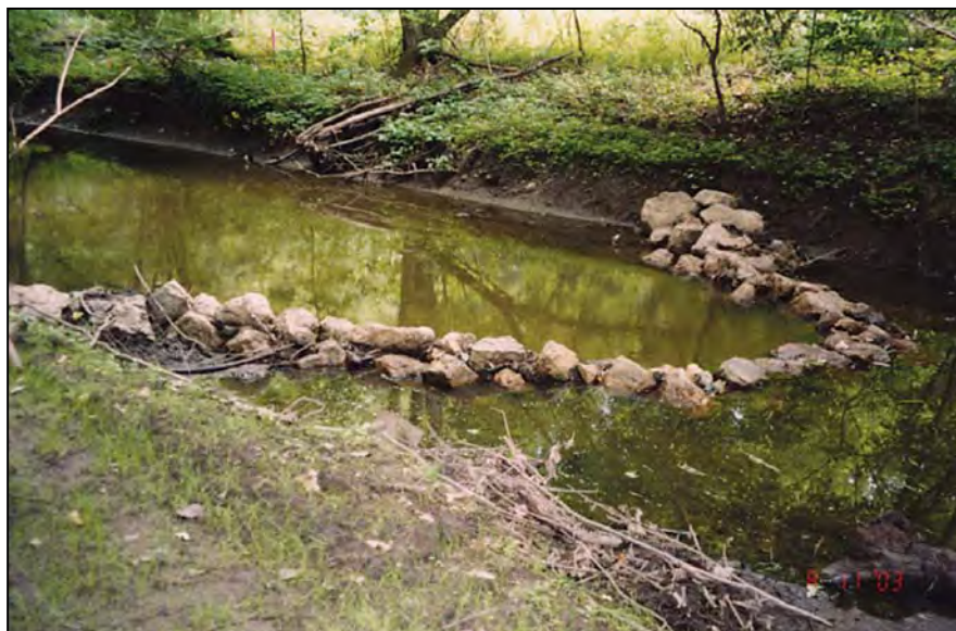
Cross-Vane in Carrier Creek, Eaton County
