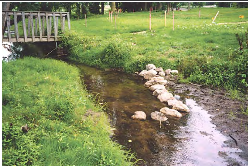
J-hook-Vane in Carrier Creek, Eaton County
