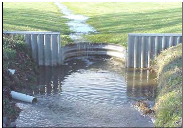
Sheet metal piling structure with weir and wing walls.
