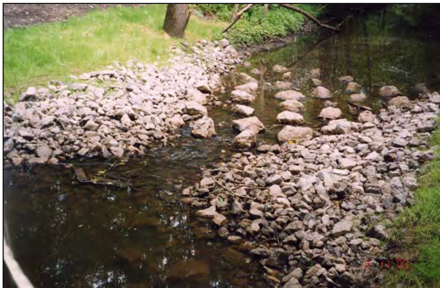
Riffle Zone installation in Carrier Creek, Eaton County
