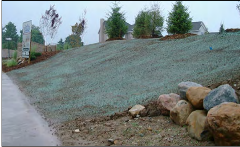
Seed, mulch and spray soil binding polymer applied prior to 1 inch rainfall in October 2001.
