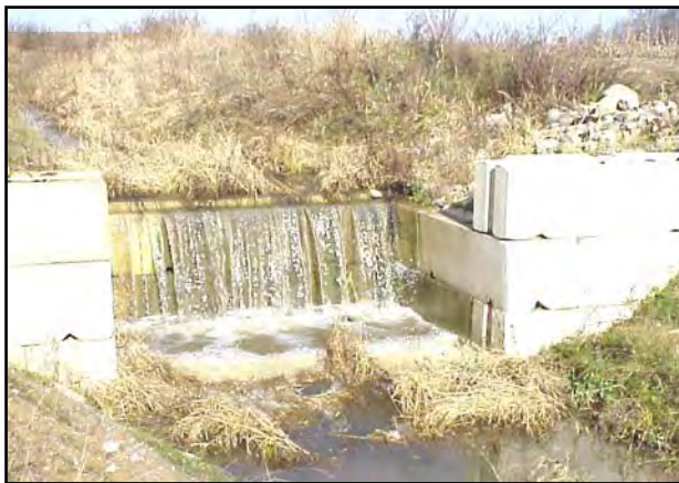
Concrete waste-block structure with weir and wing walls.
