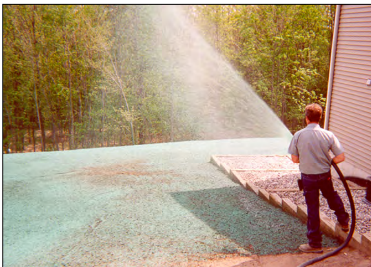
Soil binding polymer and seed being applied with hydroseeding equipment.
