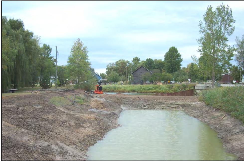
Sheet piling is being used to isolate a drain outlet from the Saginaw Bay during a drain reconstruction project.
